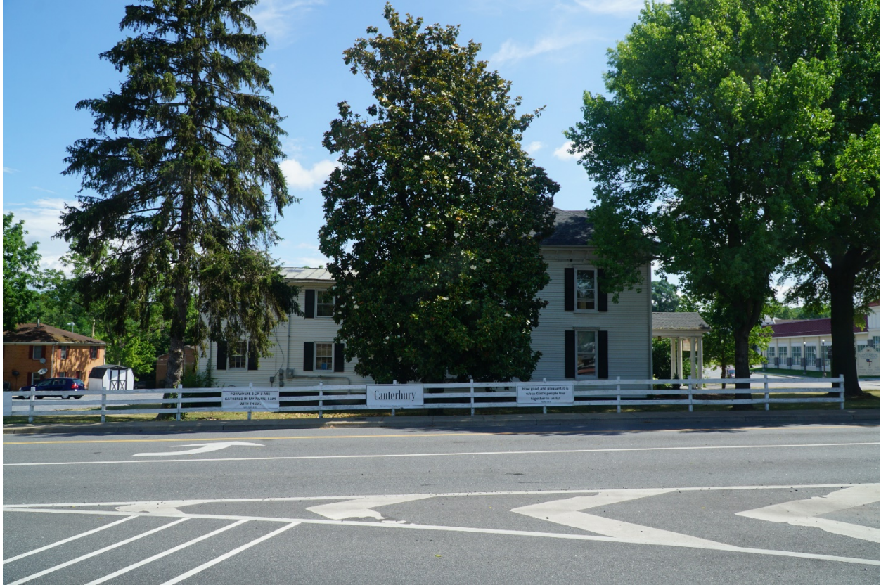
Photo 8: 741 South Main Street, Harrisonburg, VA. South Elevation, view to north. 14 July 2021.
