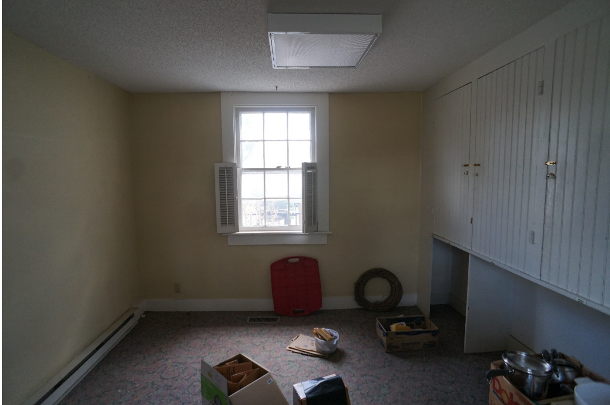
Photo 34: 741 South Main Street, Harrisonburg, VA. First Floor, back room (ell), view to north. 14 July 2021.
