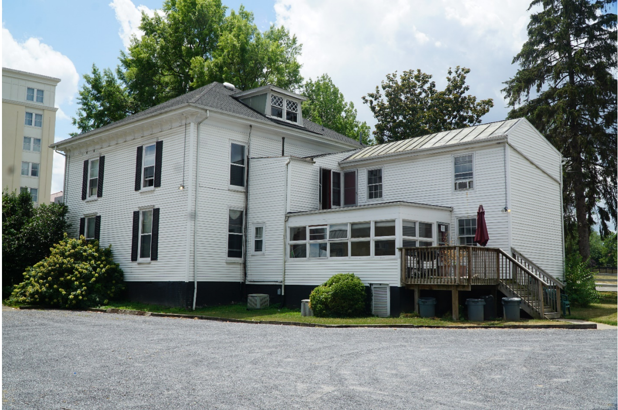
Photo 14: 741 South Main Street, Harrisonburg, VA. North Elevation, view to southeast. 14 July 2021.
