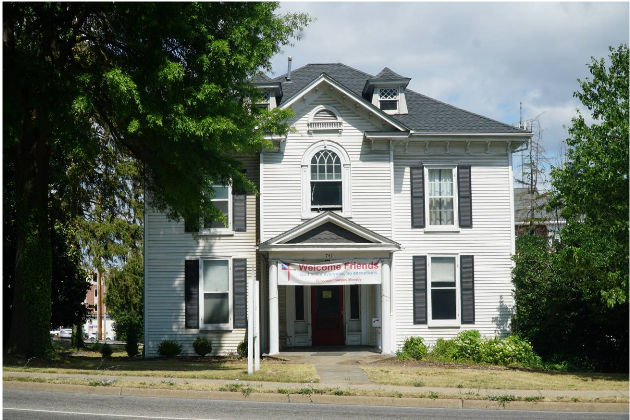
Photo 1: 741 South Main Street, Harrisonburg, VA. East Elevation (primary), view to west. 14 July 2021.
