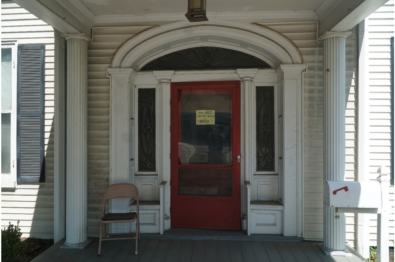
Photo 2: 741 South Main Street, Harrisonburg, VA. East Elevation (primary), view to west. 14 July 2021. Detail of entry.
