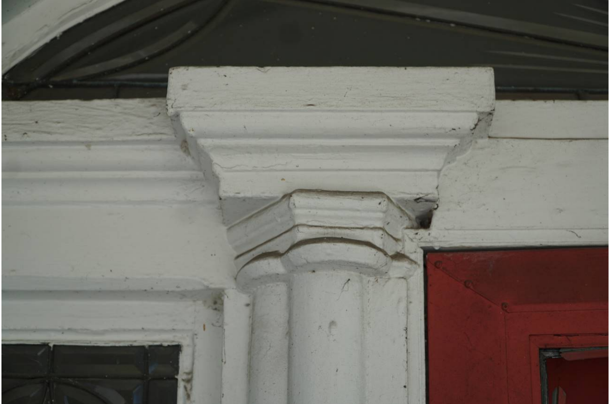
Photo 4: 741 South Main Street, Harrisonburg, VA. East Elevation (primary), view to west. 14 July 2021. Detail of compound engaged column at entry door.
