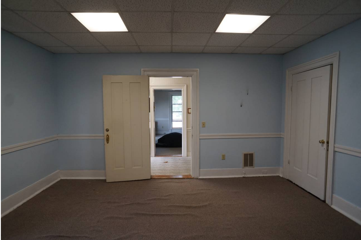
Photo 39: 741 South Main Street, Harrisonburg, VA. Second Floor, NE room, view to south. 14 July 2021.
