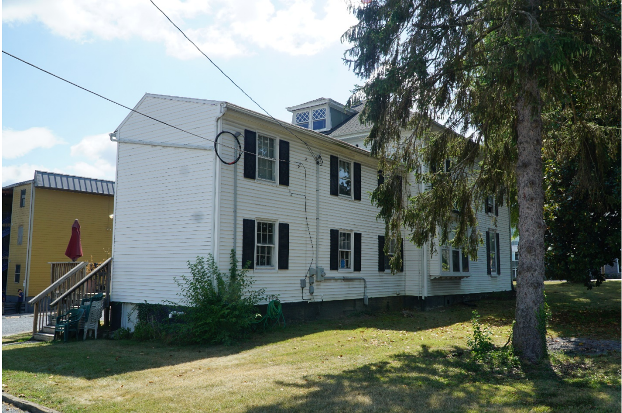
Photo 9: 741 South Main Street, Harrisonburg, VA. South Elevation, view to northeast. 14 July 2021.
