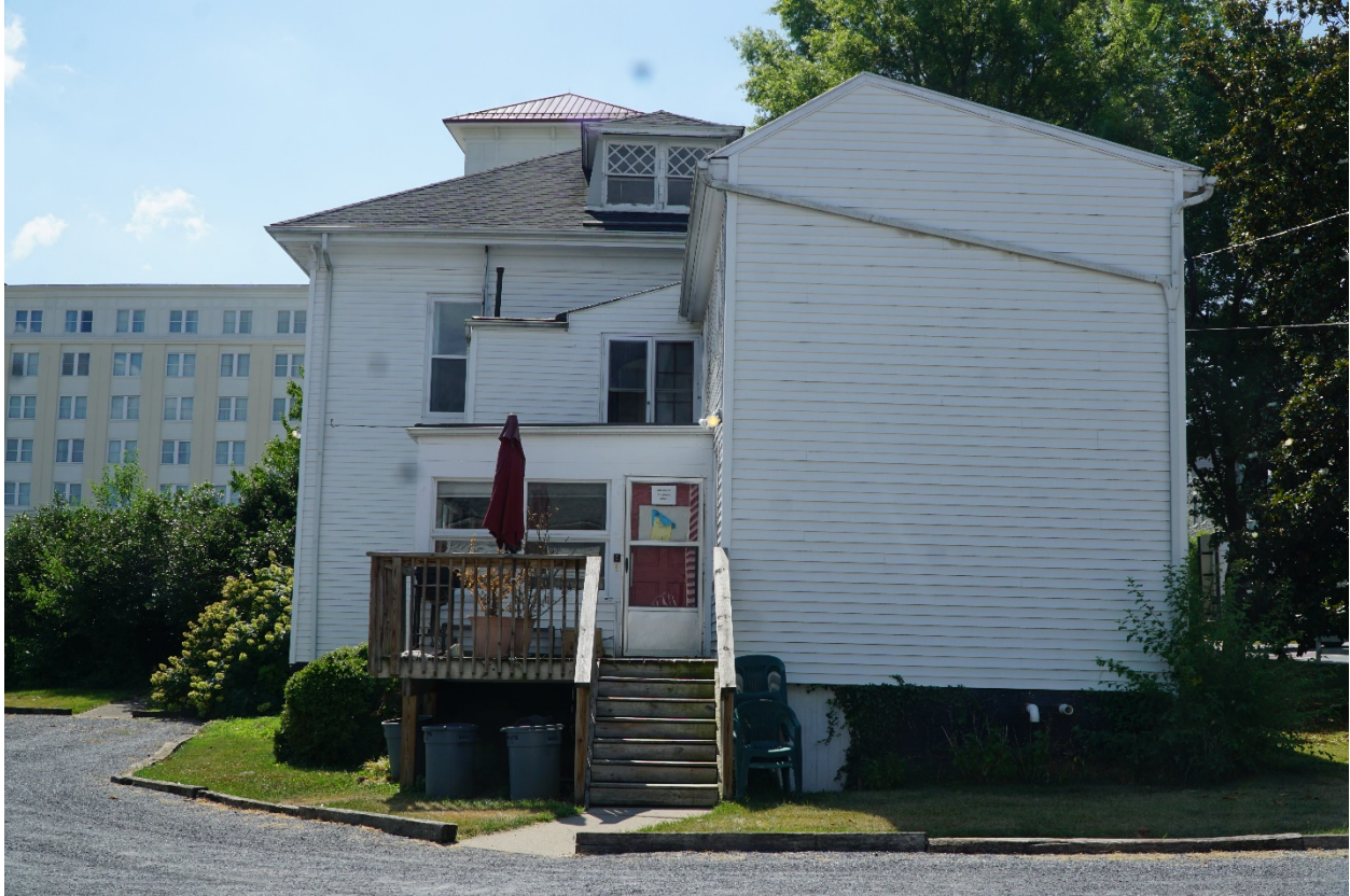
Photo 11: 741 South Main Street, Harrisonburg, VA. West Elevation, view to east. 14 July 2021.
