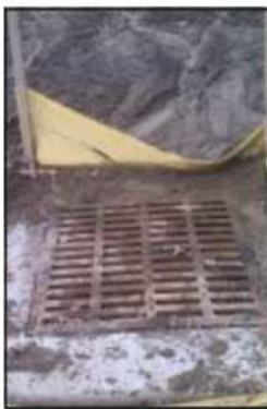
Standard drop inlet grate.
