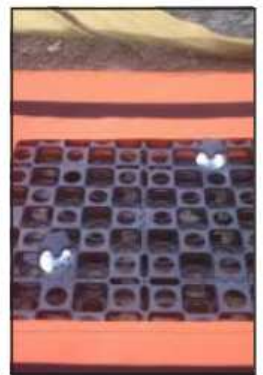
Install safety caps on anchors.
