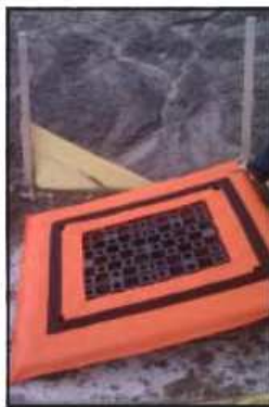
Install Grate Pyramid base over grate.
