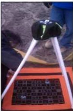
Install tower frame.
