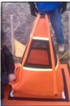
Slide tower filter over frame.
