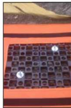
Install base with 2 to 4 anchors as needed.
