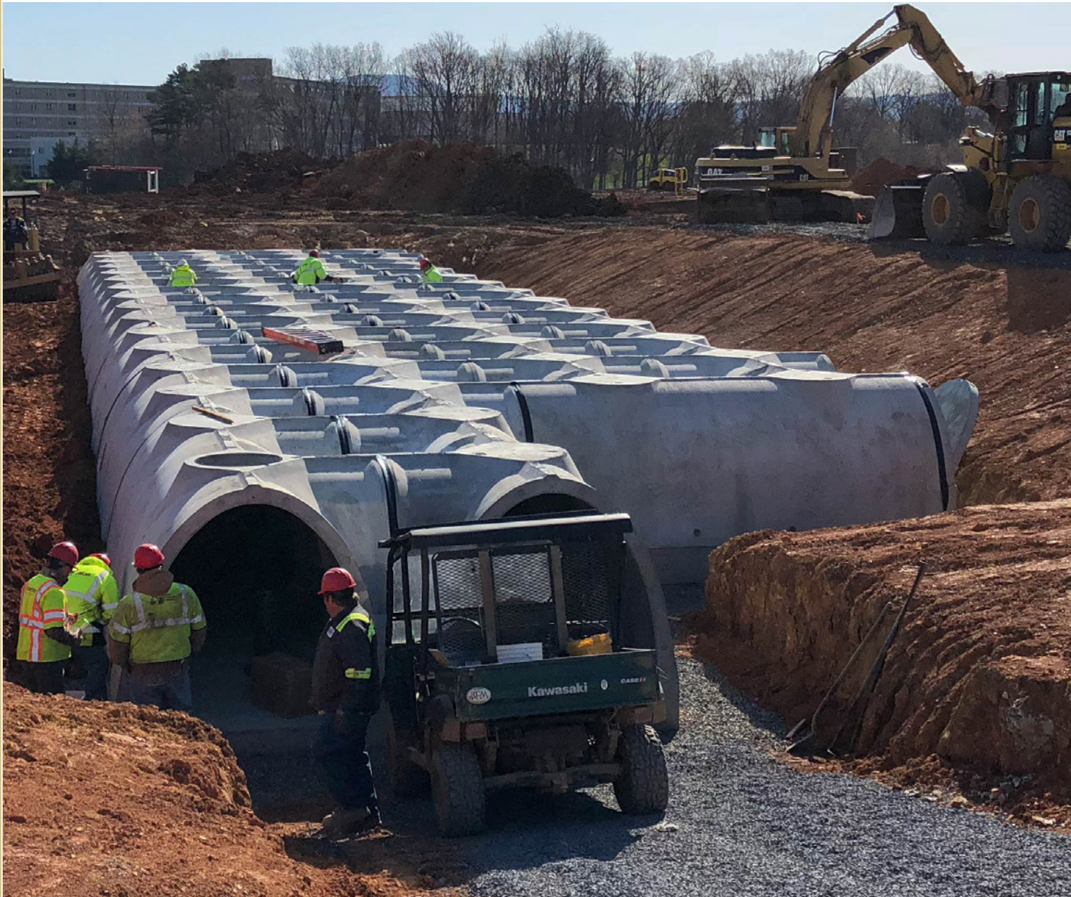
Installation of Underground Detention at Jennings Hall
