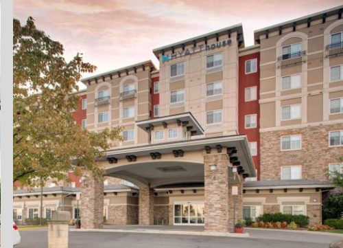
HYATT House Sterling/Dulles Airport 45520 Dulles Plaza, Sterling, VA
